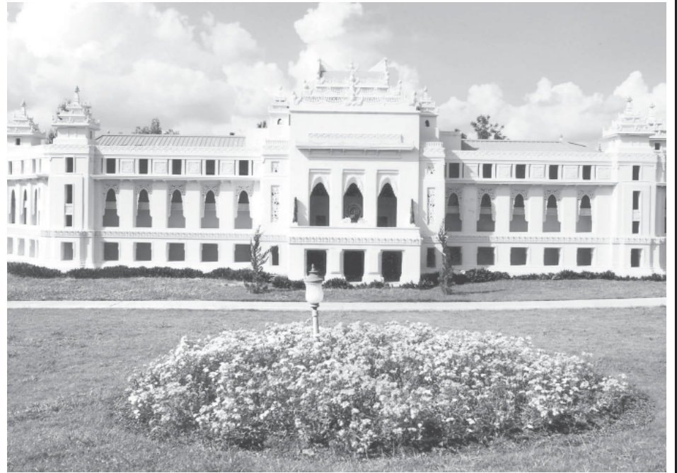
Replica of Yangon City Hall built by Htoo Trading Co Ltd.
