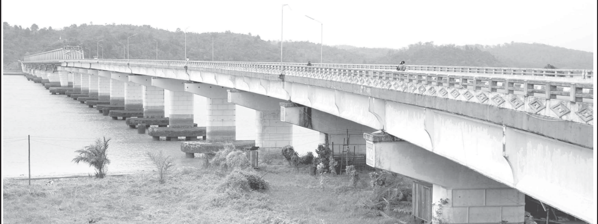
A view of 3612-foot Kyweku-Kyaukphya Bridge linking Kyweku and Kyaukphya Villages in Myeik Township, Taninthayi Division.
