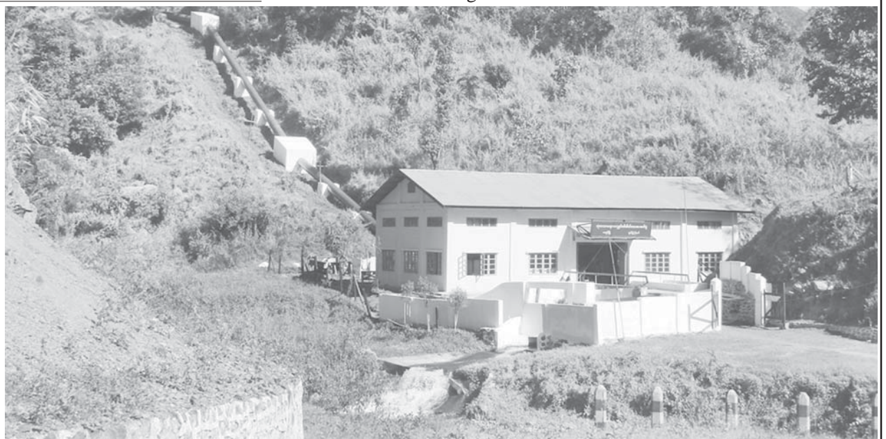
Bontalar Hydropower Station is six miles from Matupi.
