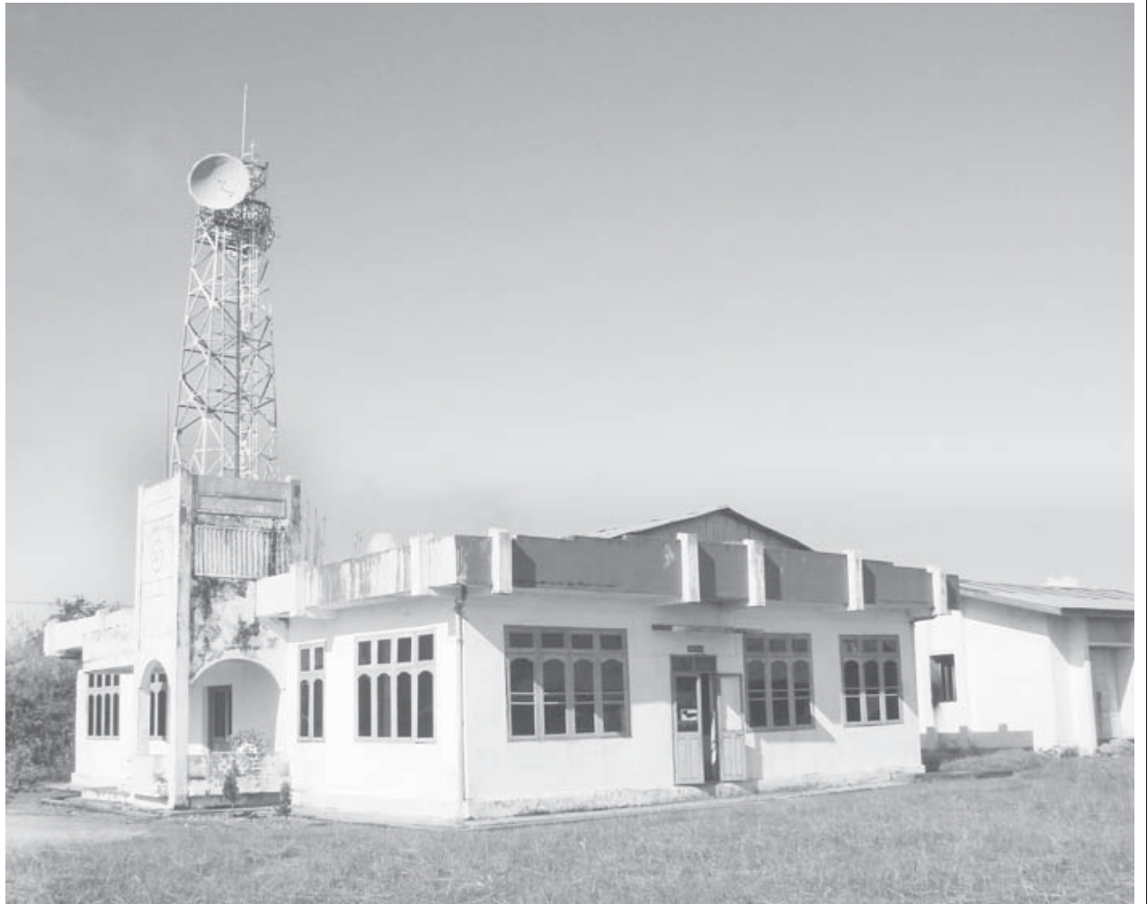
The Myanma Posts and Telecommunications (Falam branch).
