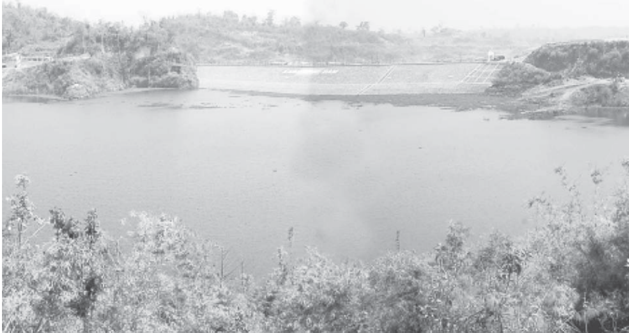
Khabaung Dam for agricultural and power generation purposes.
