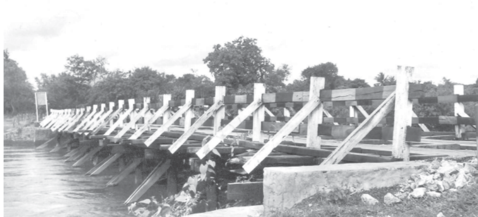
Dawei-dan Bridge, which contributes towards smooth transport of Kayin State.
