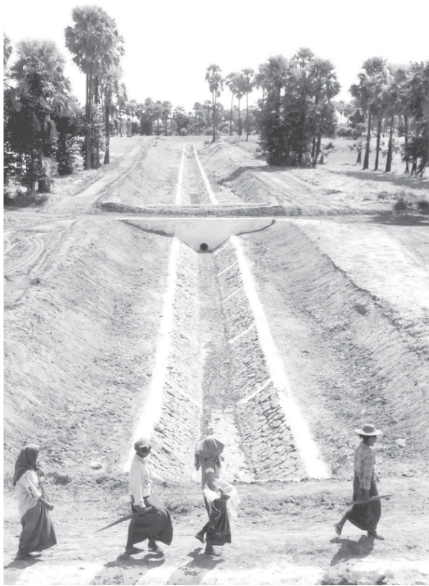
Sabay Dam, 6,900 feet long and 32 feet high, built near new Sabay Village in Pakokku Township.
