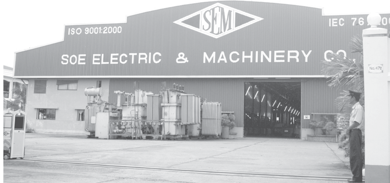
Transformer Factory of Soe Electric & Machinery Co Ltd seen in Dagon Myothit (South) No. 1 Industrial Zone. —MNA
