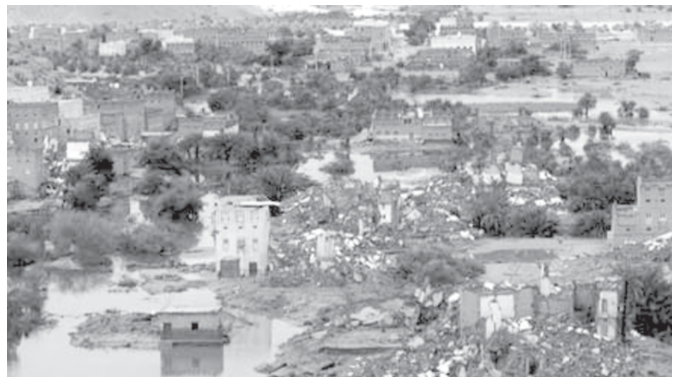
Houses damaged by floods are seen in the eastern province of Hadramout, Yemen, on 25 Oct, 2008. — XINHUA
