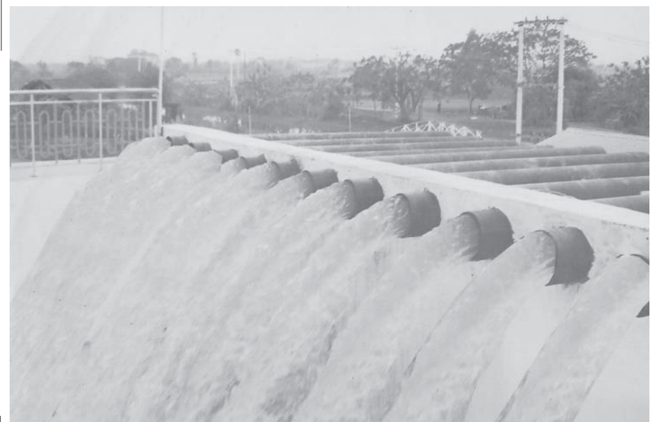
Hsinphon River Water Pumping Station irrigating 37,000 acres of summer paddy plantations in Hlegu Township.
