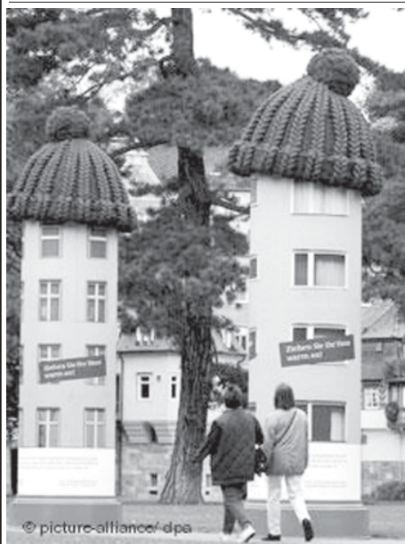
As Germans start stoking their heating systems in anticipation of the annual winter chill, the federal interior ministry advised property owners to "dress their buildings warm for winter." A display of nine columns topped Trevira fibers made to look like wool caps began its tour around Germany in the southern German city of Esslingen. The ministry said the display is intended to promote environmentally friendly building refurbishment.
