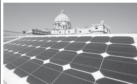
St Peter's Basilica is seen behind a solar panel set up on the roof of the Paul VI Hall, at the Vatican. According to workers involved in the project, a total of 2,700 panels will be placed at the Vatican to provide 300,000 kilowatt hours of electricity to be used to illuminate, heat or cool the building where the pontiff holds general audiences in the winter and bad weather as well as concerts.
