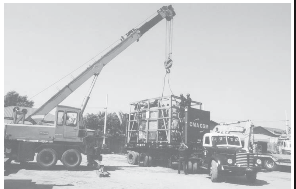
Heavy machinery being operated in the worksite of Yangon Transformer Factory.
