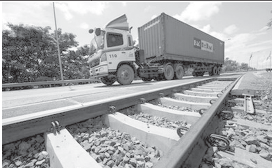
A truck drives past railway tracks at the Thai-Laos Friendship Bridge in Nong Khai province near the Thai-Laos border, in August.—INTERNET
