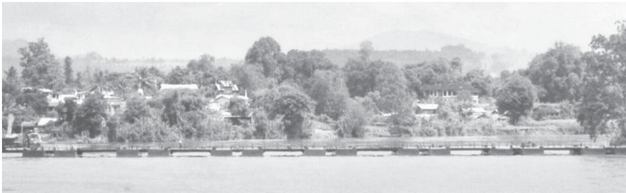
Photo shows downstream view of Dokhtawady River Pontoon Bridge on 6 September.
