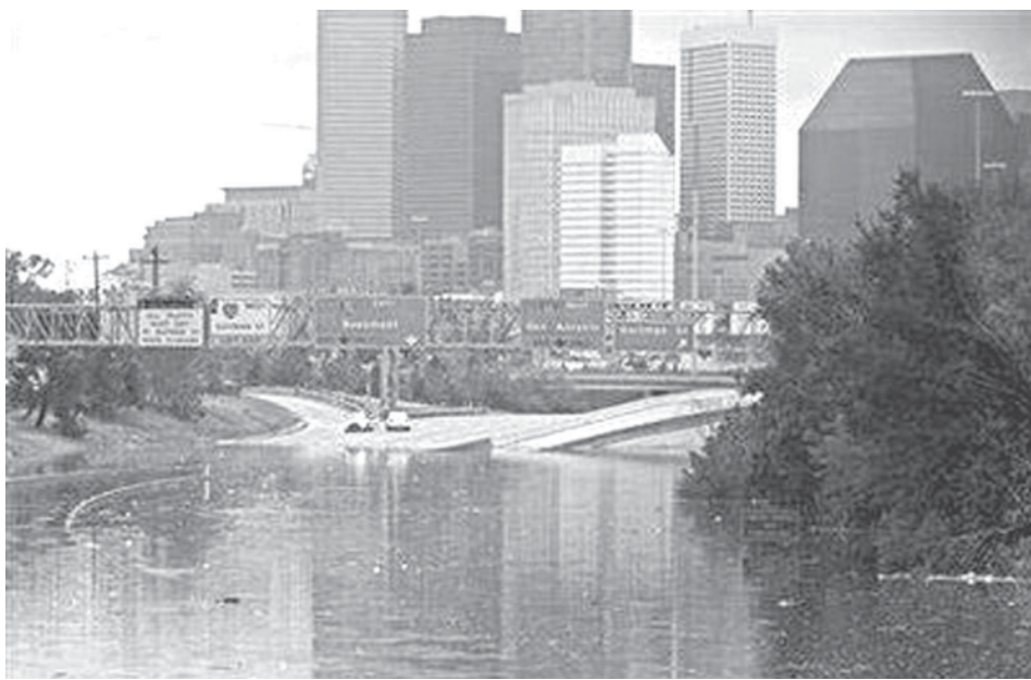
Interstate 45 leading into downtown Houston is blocked by police after the major transportation artery was closed by flooding caused by rains following Hurricane Ike September 14, 2008.—REUTERS
