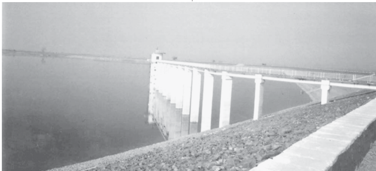
Water control tower of Ma Mya Dam.
