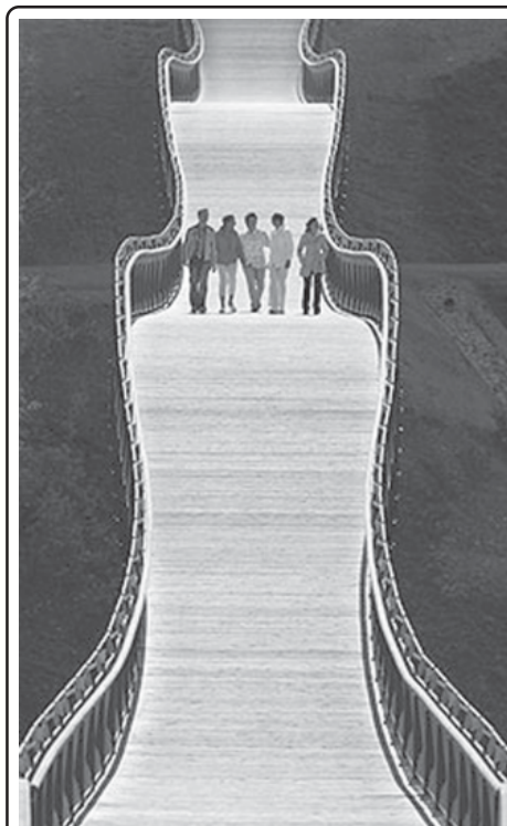
Serious Span Europe's longest wooden bridge spans a valley of the 2007 Bundesgartenschau (German Federal Garden Show — BUGA) area in Ronneburg near Gera, eastern Germany. The bridge is 787 feet long.
