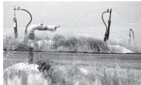
Pipes that extract methane gas generated by waste decomposition are seen at the Simi Valley Landfill and Recycling Center in Simi Valley, California on 8 May, 2008. —INTERNET
