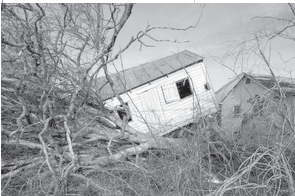
A view of a house thrown from its foundation by Hurricane Ike, on Great Inagua Island, in the southern Bahamas, on 9 Sept, 2008. Ike was a category 4 hurricane as it passed over Great Inagua on 7 Sept. —INTERNET
