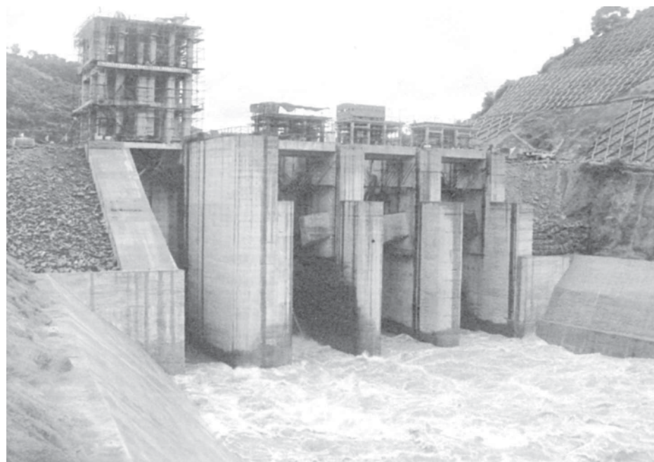
The concrete works of main embankment at the hydropower project.
