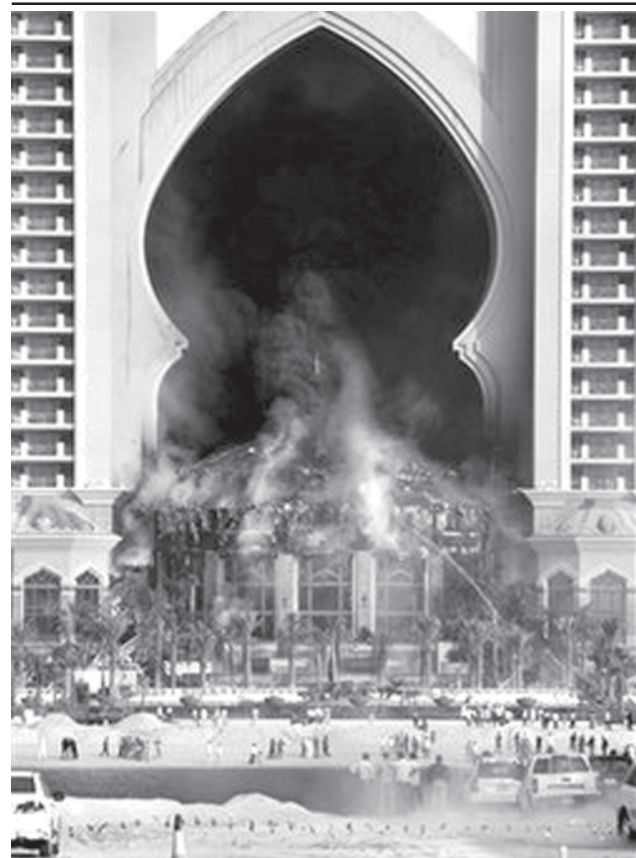
A fire burns in the five-star Atlantis hotel, which was set to open later this month and currently has no guests in it, on the man-made Palm Island in Dubai, United Arab Emirates, Tuesday, 2 Sept, 2008. Firefighters have been battling flames in the lobby of the five-star hotel on the artificial island which was built in the shape of a palm tree, but the cause of the fire is not yet known.—INTERNET
