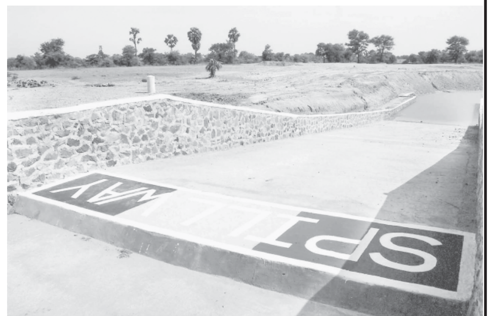
25 feet wide RC spillway seen at Kyauksauk Dam.
