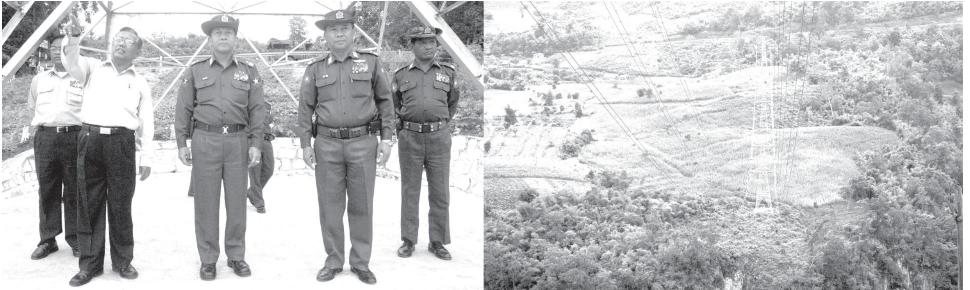
Maj-Gen Min Aung Hlaing inspects installation of Shweli-Mansan-Shwesayan 230 KV power line. — MNA
