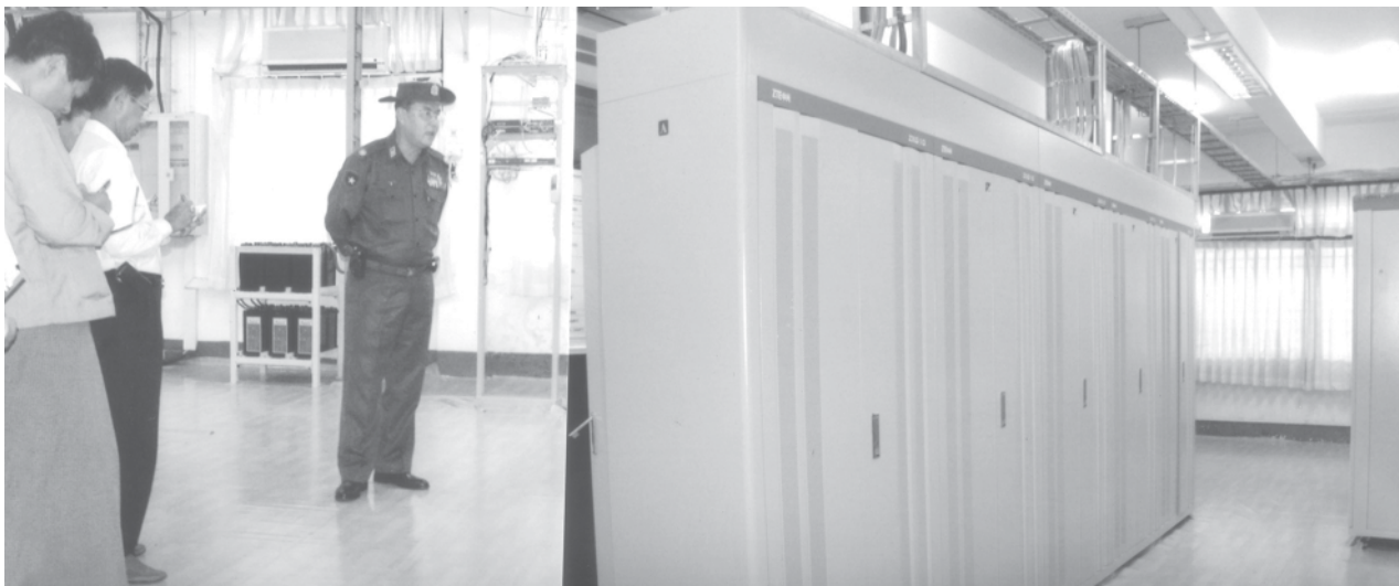
Minister Brig-Gen Thein Zaw inspects an Auto-exchange in Pyigyidagun.—MPT
