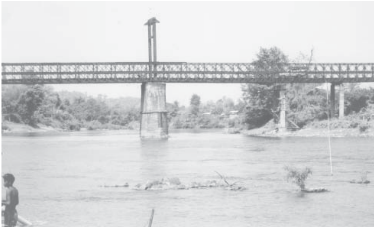
Photo shows existing Hsipaw Dokhtawady Bridge.
