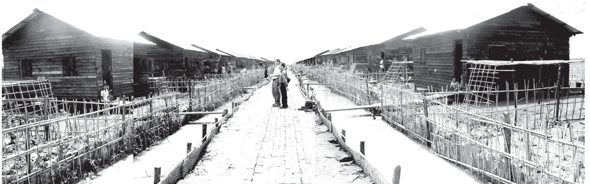
Houses for storm victims seen at Satsan village, Bogale Township.—MNA
