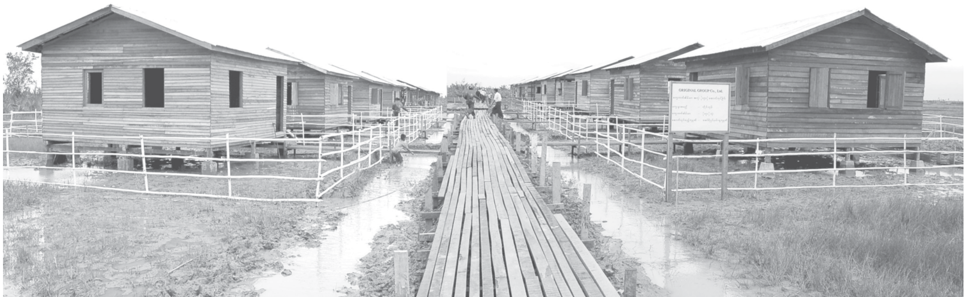
Houses built by Original Group Co for the storm victims in Hlaingbone village. — MNA
