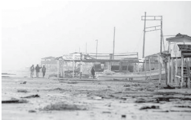
Residents walk on a debris-covered beach near buildings damaged by Hurricane Dolly on Bagdad beach, some 38 km (24 miles) from the border city of Matamoros on 24 July, 2008. After Hurricane Dolly unleashed a fury of damaging winds and wicked rain on the US-Mexico coastline and diminished to a tropical storm, widespread flooding along the populous Rio Grande Valley became the top concern on Thursday.—INTERNET
