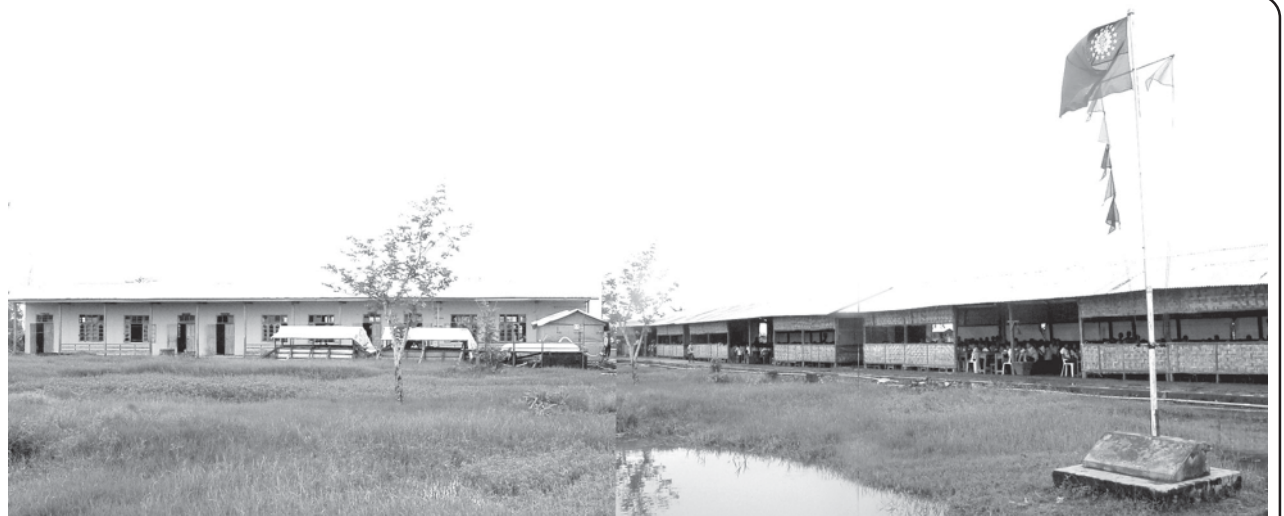
Temporary school buildings in Satsan Village in Bogale Township.—MNA
