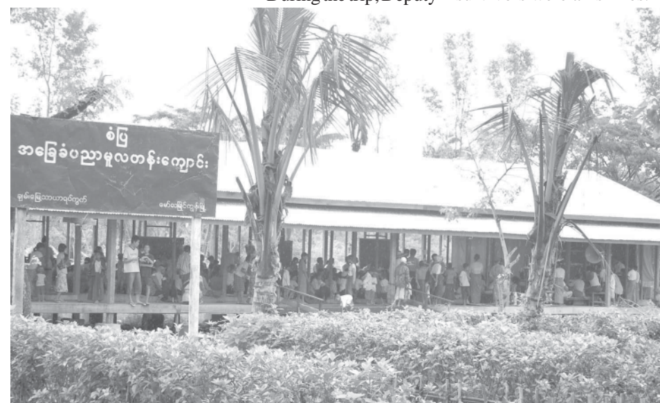
The photo shows Basic Education Primary School in Chanmyethaya Ward after being repaired.
