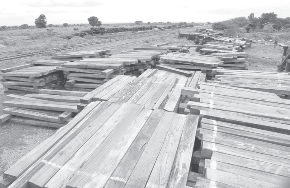
Sleepers to be used in constructing railroad.
