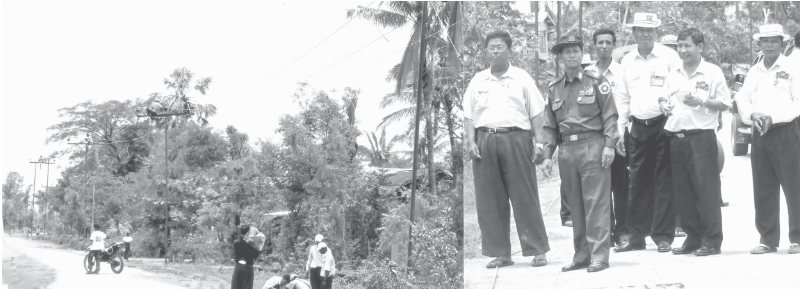
Minister Maj-Gen Khin Maung Myint observes installation of cables from Kanbe junction to Dalla Township.—EP NO. 2
