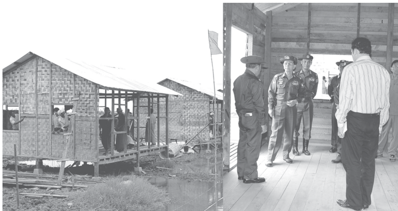
Prime Minister General Thein Sein inspects construction of houses in Kyeinchaunggyi village, Bogale Township.—MNA
