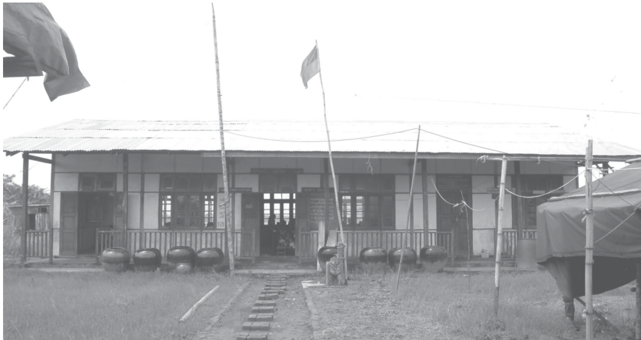
Ngatantaya Basic Education Primary School seen after being repaired.
