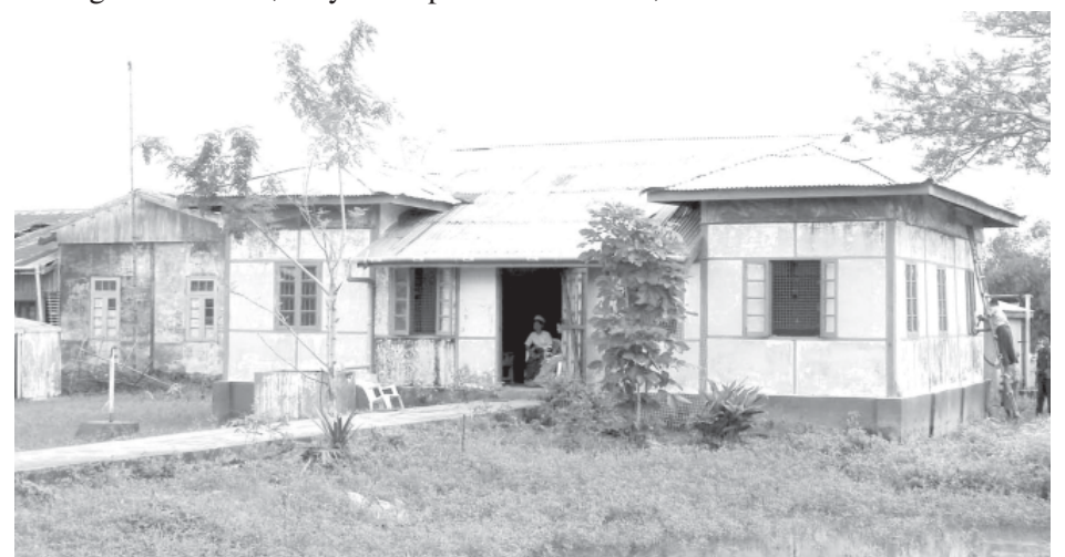
Pyinsalu People's Hospital of Ayeyawady Division seen after being repaired.
