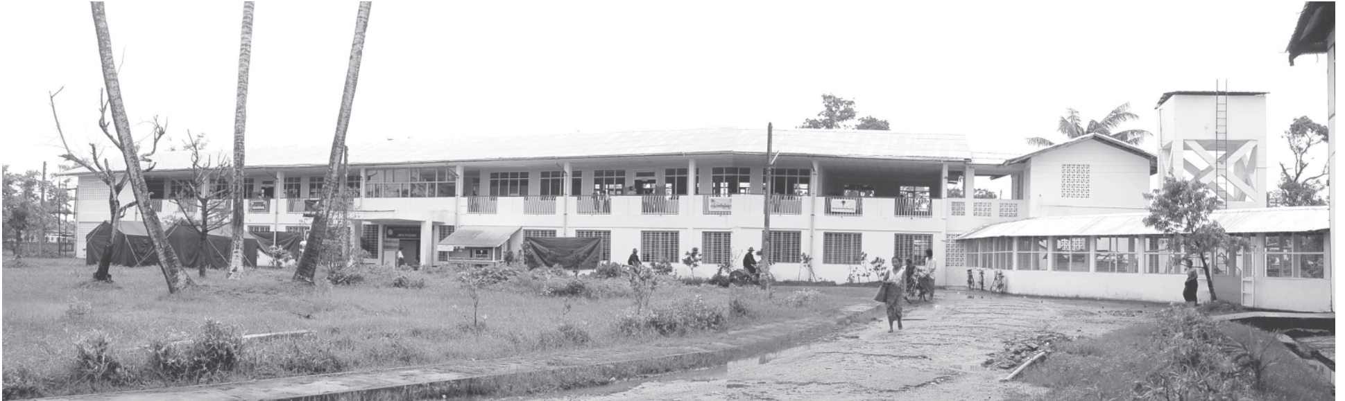
People's Hospital in Pyapon seen after being repaired. — MNA
