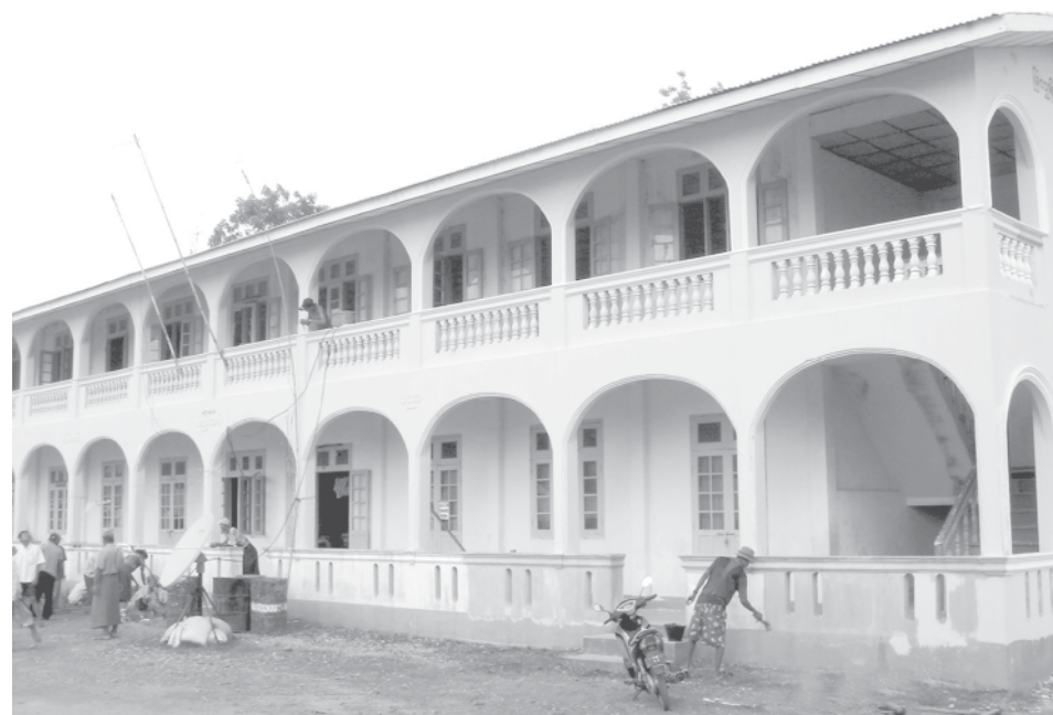
The repaired Hainggyikyun Basic Education High School.
