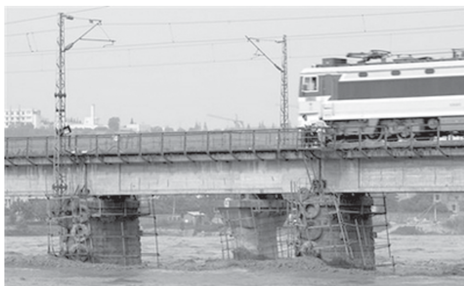
A train crosses the Chengdu-Baoji railway bridge, whose support columns are protected against floating debris, as the floodwater from Tangjiashan quake-formed lake flow down the Fujiang River in Mianyang of southwest China's Sichuan Province on 10 June, 2008.—INTERNET
