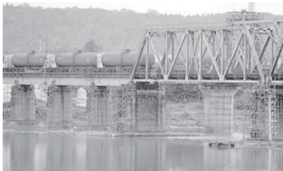
A freight train travels on a Chengdu-Baoji Railway bridge, with protected support columns, spanning the Fujiang River, which is connected to the Tangjiashan quake lake, in Fucheng district of Mianyang, Sichuan Province on 7 June, 2008. Chinese troops began easing pressure on the dangerously swollen 'quake lake' on Saturday, with water gushing into a man-made sluice in an operation monitored by satellite.—INTERNET
