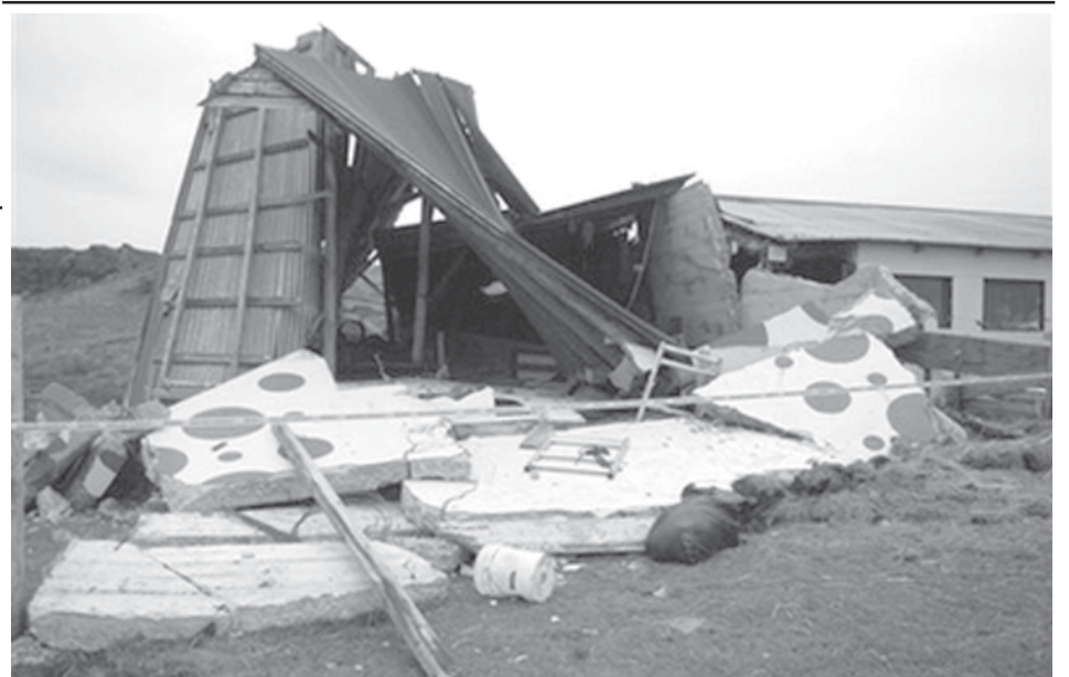
A building damaged by an earthquake is seen near the town of Selfoss in Iceland, on 30 May, 2008. A powerful earthquake shook Iceland on Thursday, rocking buildings in the capital, lightly injuring more than a dozen people and forcing residents in outlying towns to evacuate. —INTERNET
