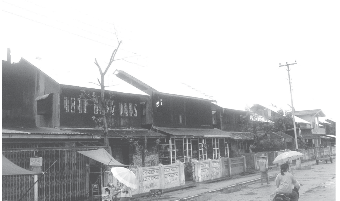
Photo shows repaired buildings in storm-hit Bogale Township. — MNA
