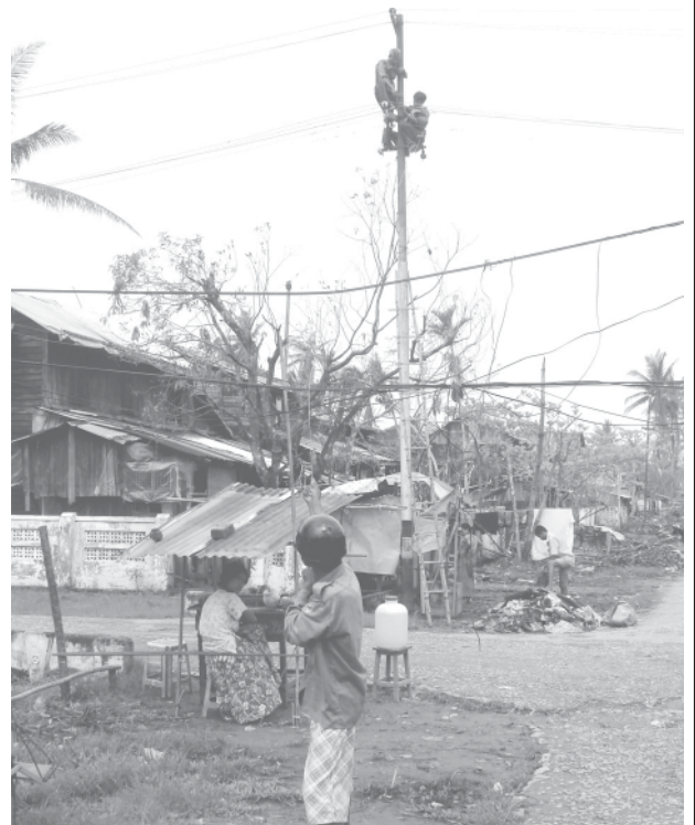
Electricians repair cables in Bogale.—MNA
