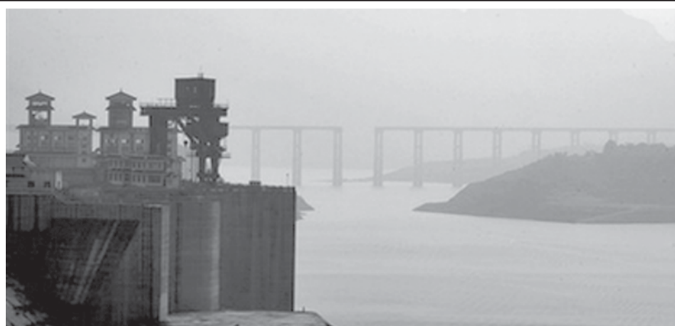
The Zipingpu Dam buildings are seen at left near a bridge where the middle section is fallen after Monday's earthquake near Dujiangyan, southwestern China's Sichuan Province, on 15 May, 2008. China warned the death toll from this week's earthquake could soar to 50,000, while the government issued a rare public appeal Thursday for rescue equipment as it struggled to cope with the disaster.—INTERNET
