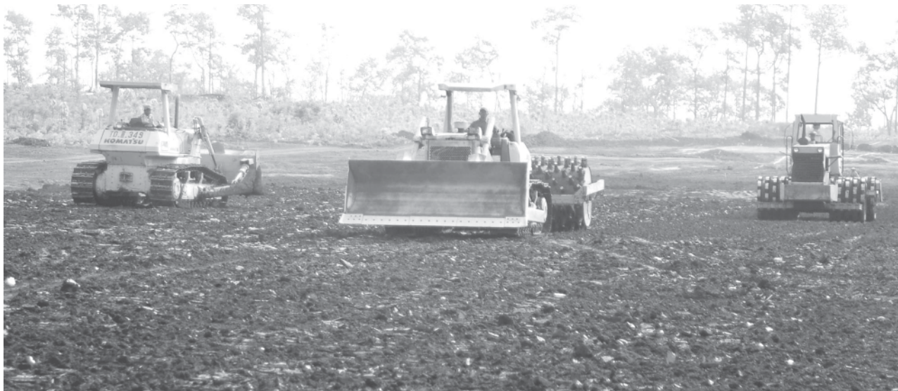
Construction task of Kyaingkham Dam by heavy machinery in Yaksawk Township.—MNA
