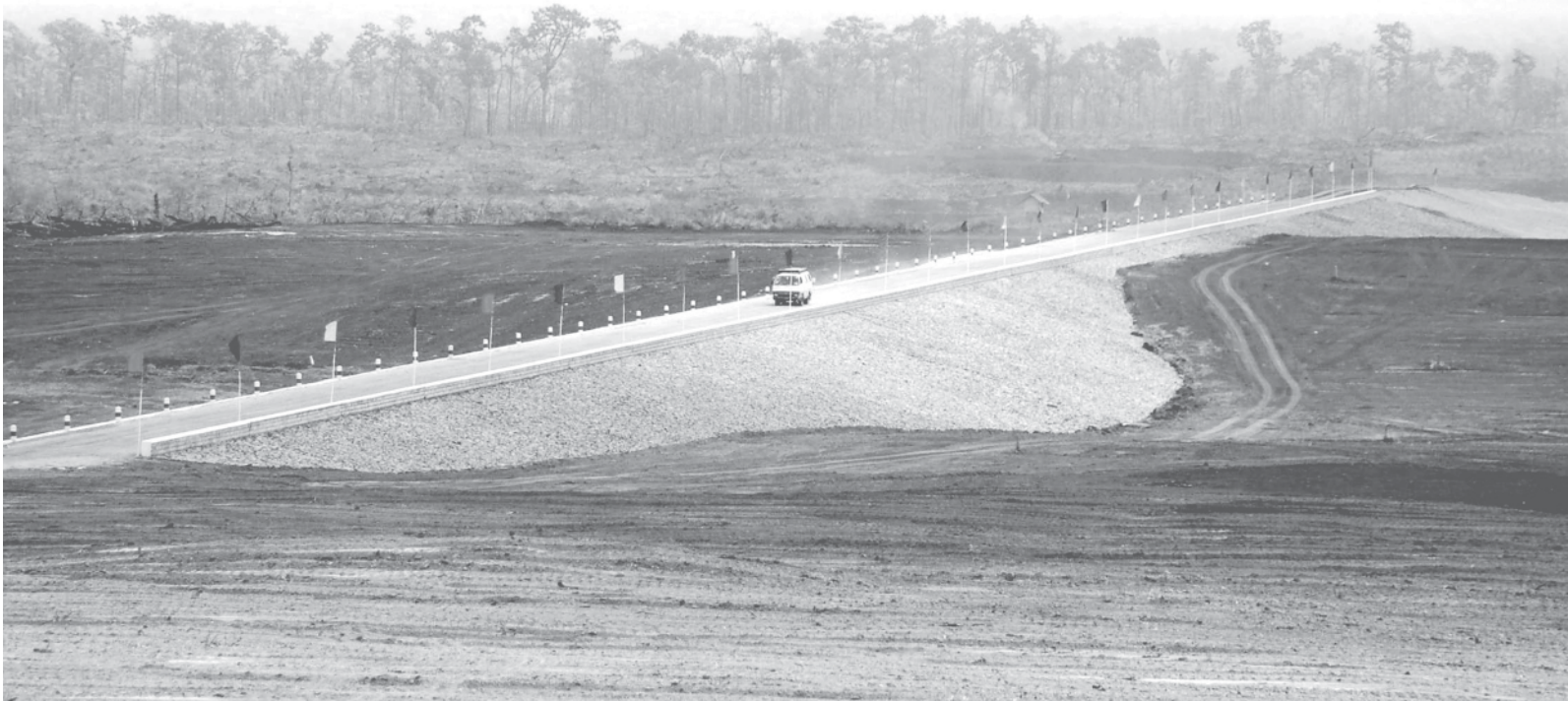
Kyaingkhram Dam under construction in Yaksawk Township.—MNA
