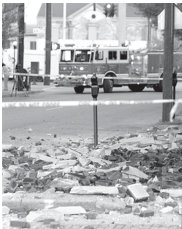
An emergency vehicle waits at the scene where rubble from earthquake damage lies strewn along a sidewalk in an old section of Louisville, Ky, on 18 April, 2008. The 5.2 magnitude earthquake, centered in southern Illinois, rattled skyscrapers in Chicago's Loop and homes in Cincinnati but appeared to cause no major injuries or damage.—INTERNET
