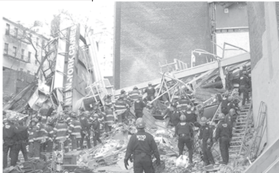
Rescue workers work at the scene of a crushed building on 50th Street near Second Avenue Saturday, on 15 March, 2008 in New York. A giant crane toppled over at a construction site and smashed into a block of residential killing four people and setting off a scramble for survivors.
