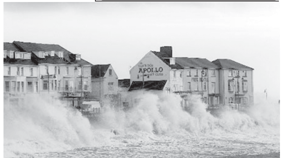
Waves hit the sea wall in Porthcall, south Wales on 10 March, 2008. A storm rushing in from the Atlantic lashed the south west on Monday as high winds and tides brought the risk of coastal flooding.—XINHUA
