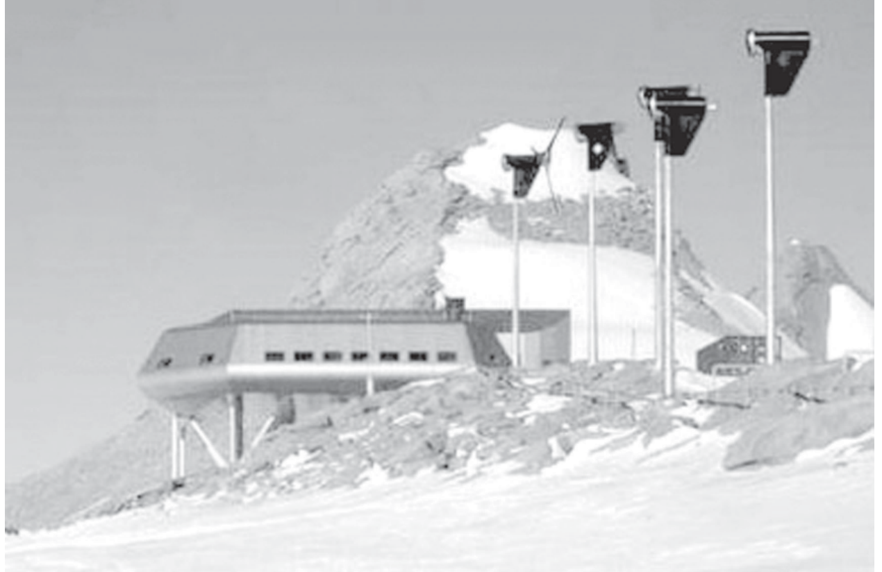
View of the Belgium’s Princess Elisabeth polar station, received at a news conference on the first phase its construction, in Brussels March 11, 2008. Belgium is building the first ever zero-emission polar station in the Antarctic, powered by solar panels and wind turbines and designed to have minimal impact on the climate change its scientists are studying. —INTERNET
