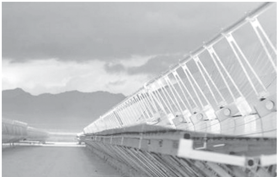
Mirrors are seen channelling sunlight onto a tube filled with oil during the dedication of Acciona's Nevada Solar One power plant in Boulder City, about 30 miles (48 kms) southeast of Las Vegas on 22 Feb, 2008. Acciona is a renewable energy company based in Spain. —INTERNET
