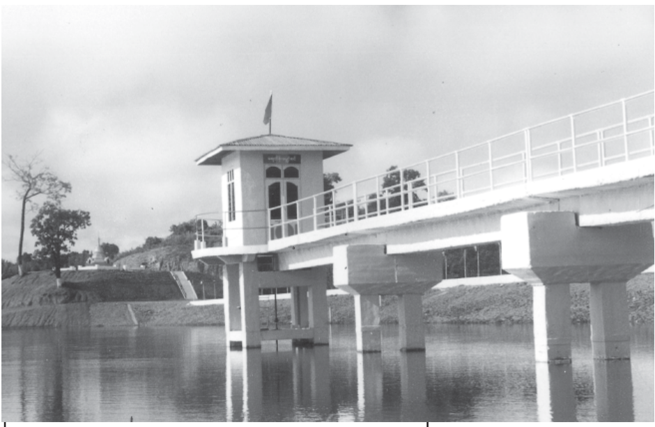
With the aim of supplying water to arable lands and local people Hinywet Dam was built in An Township of Rakhine State.
