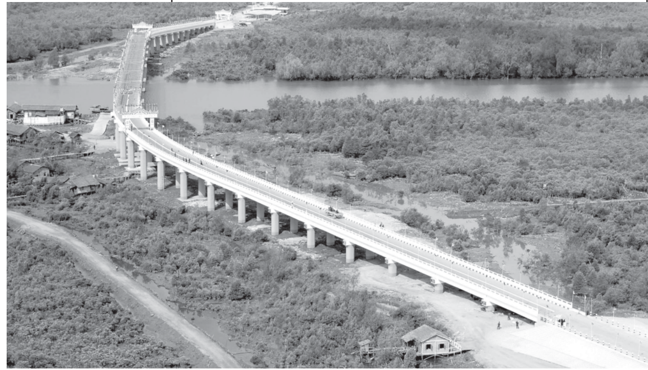
The photo shows Minkyaung Creek Bridge constructed on Yangon-Sittway Highway in Rakhine State.
