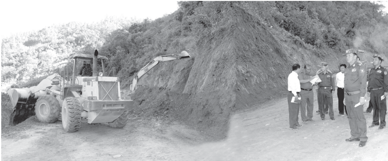
Maj-Gen Khin Zaw inspects roadworks at Haka-Gangaw road section.—MNA
