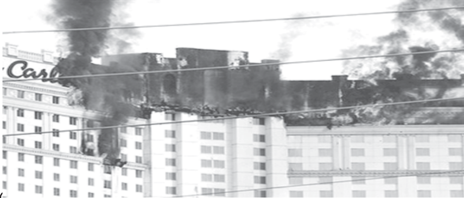
Smoke and flames rise after a fire broke out at the Monte Carlo hotel-casino in Las Vegas, Friday, on 25 Jan 2008. The fire, which was reported around 11 am, Friday halted gambling at the casino as it spread from the center of the building across the roof. No major injuries were reported, said Clark County spokesman.
