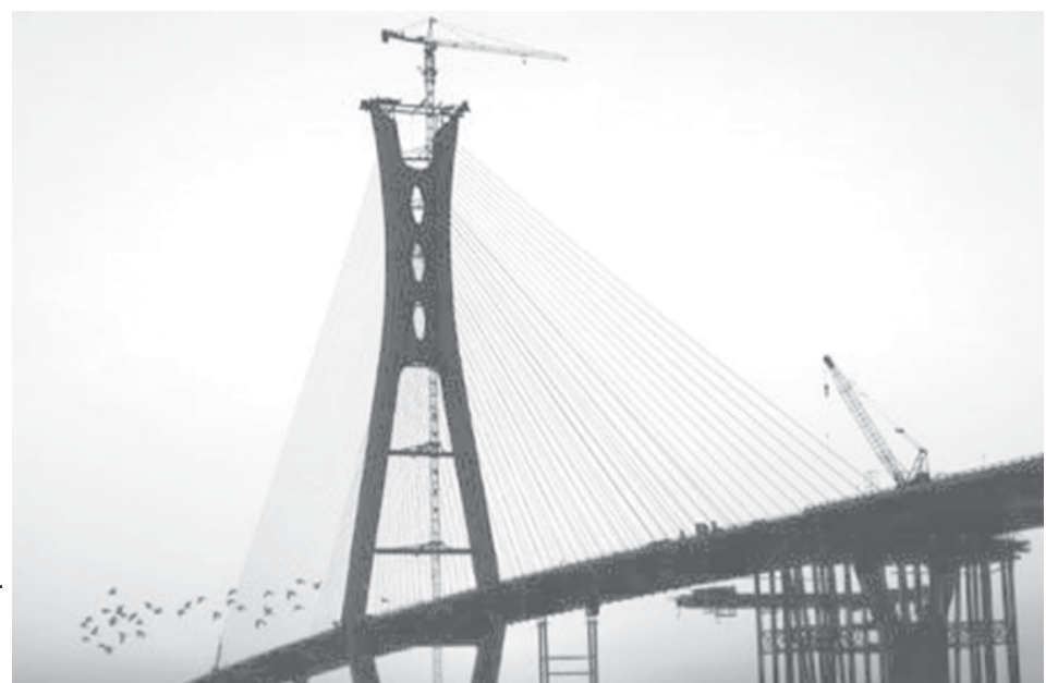
A 3 kilometre long, 33 metre wide bridge in Rui’an City, in eastern China’s Zhejiang Province, is completed on 2 Jan, 2008, after the two sections of the bridge met in the middle. The Rui’an Bridge, a two-way road with six lanes, has a weight capacity of 3,000 tons.—INTERNET
