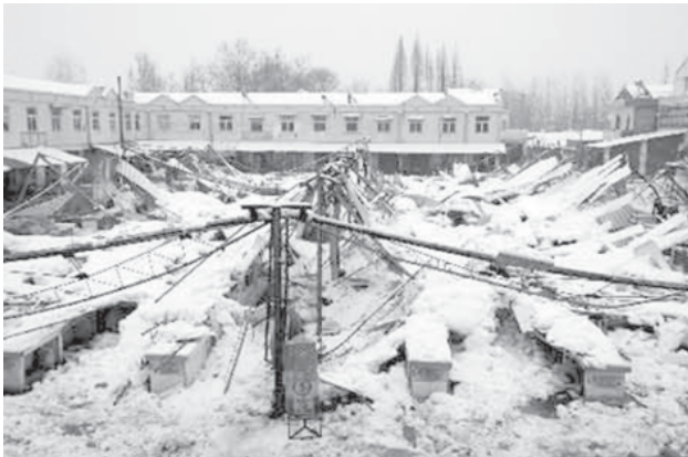
The heavy snow covers a collapsed building in a market in Shucheng county of east China's Anhui Province, on 22 Jan, 2008. —XINHUA
