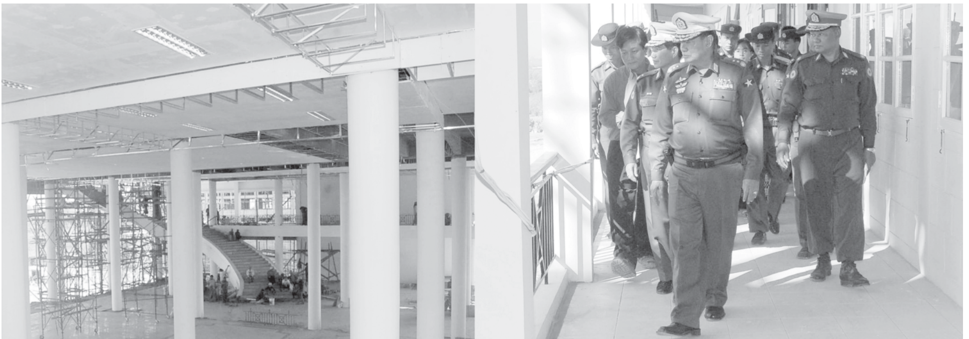
Lt-Gen Kyaw Win of Ministry of Defence inspects construction of Loikaw Technological University. — MNA
