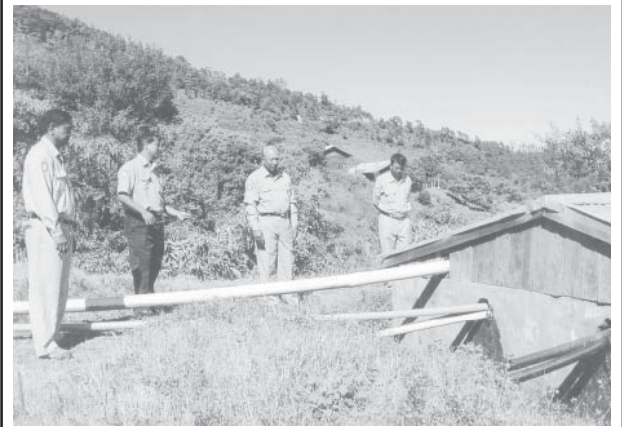
Executive Officer U Tin Oo Lay briefs U Aye Cho, Deputy Superintending Engineer of Bago Division Development Affairs Committee, on progress of earth work and designation of axis being implemented by DaikU Township DAC during 2007-2008 fiscal year. — TOWNSHIP DAC
