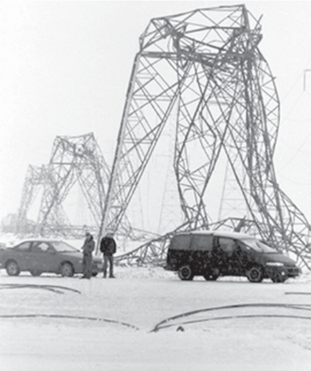
People look at a series of Hydro-Quebec high voltage towers near St-Bruno, Que, south of Montreal that collapsed after a severe ice storm hit southwest Quebec.—INTERNET
