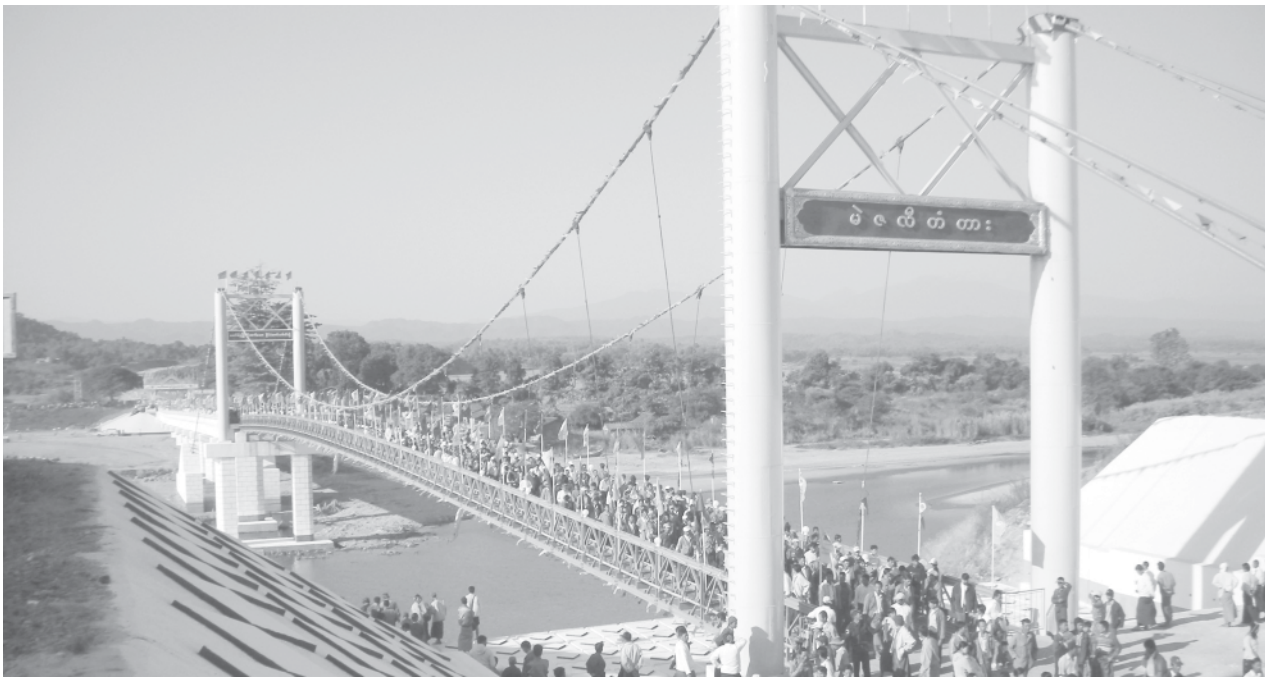
Mezali Bridge in Pwintbyu Township, Minbu District. — MNA
