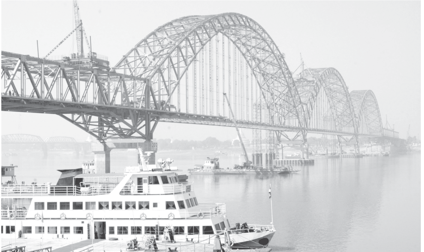
Ayeyawady Bridge ( Yadanabon ) under construction.— MNA
