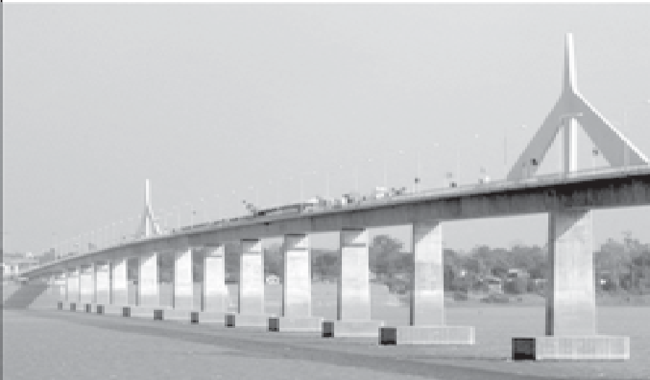
A view of the Thai-Laos second Friendship Bridge over Mae Kong River in Mukdahan Province, near the Thai-Laos border. The 1,600 meters long and 12 metres wide bridge was started in December 2003 for a cost of 2.67 billion baht (76.28 million USD).—INTERNET
